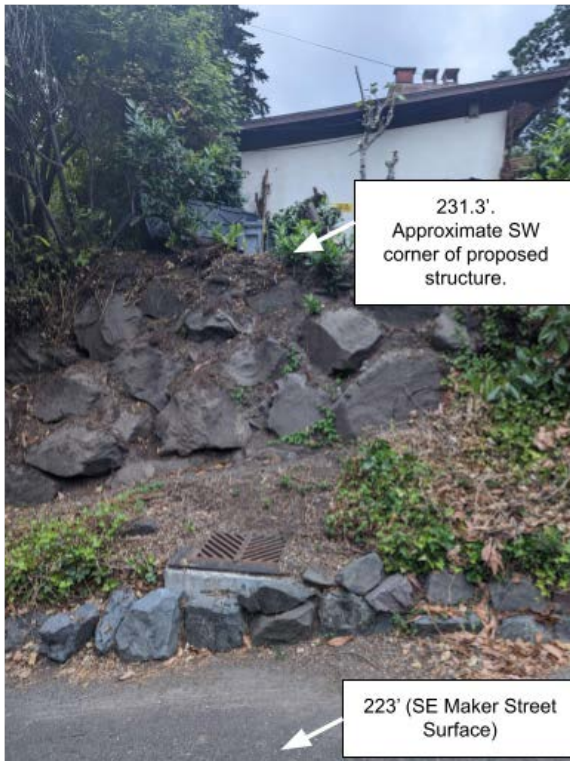
Figure 1: Retaining Wall between 6950 SE Maker Street and SE Maker Street
